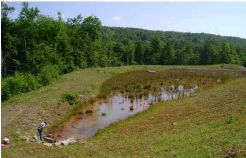
Passive Wetland Treatment System: Lausanne Tunnel water flows through pipes (forefront) into Wetland A
